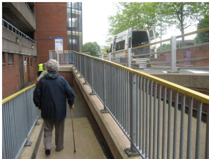
Figure 2: Dial a Ride customers access Shopmobility using a ramp located immediately beside the vehicle stopping point. The ramp uses an “anti-slip” surface which is designed to minimise the risk of customer falls.
